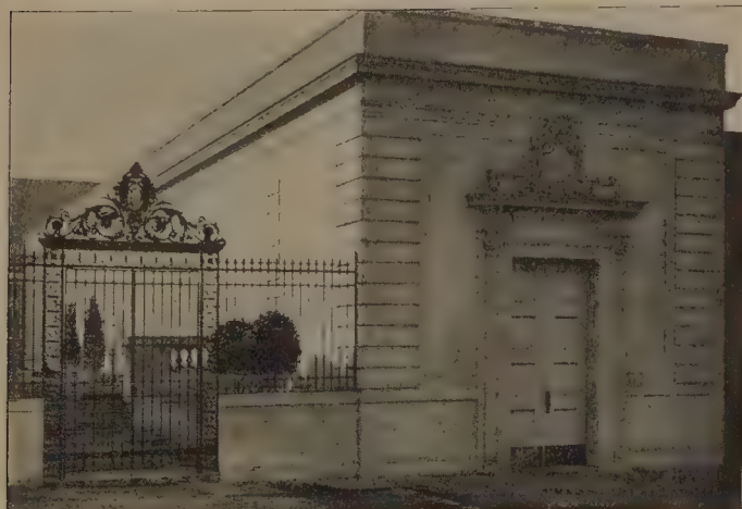
635 Willis Polk and Company, architects; photograph by Gabriel Moulin
